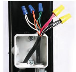
**IMPORTANT: The length of the extension cable should be as short as possible. Cable should be installed in conduit from control box to junction box.**
